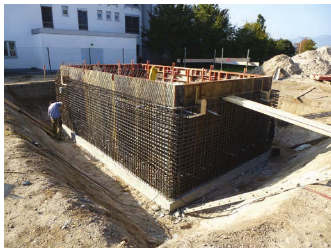
ABOVE: THE FOUNDATIONS TAKE SHAPE NEXT DOOR TO TRE'S EXISTING FACILITY IN NEUSTADT
